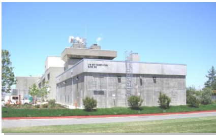
◀ SRWTP's Electrical Substation
